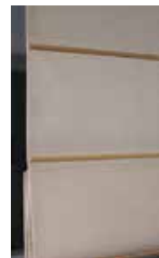
Timber Battens Front
